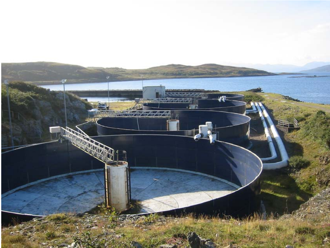
Figure 10. Land based pump-ashore marine finfish farm (currently unused). Photo courtesy of Richard Slaski
