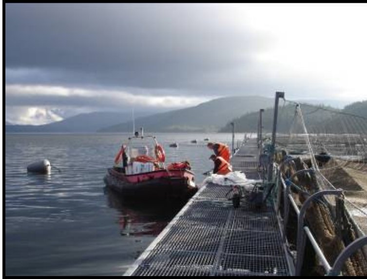
Figure 3: Walkway design and net stanchions for square steel cage design (at Camas Glas fish farm on Loch Sunart).
