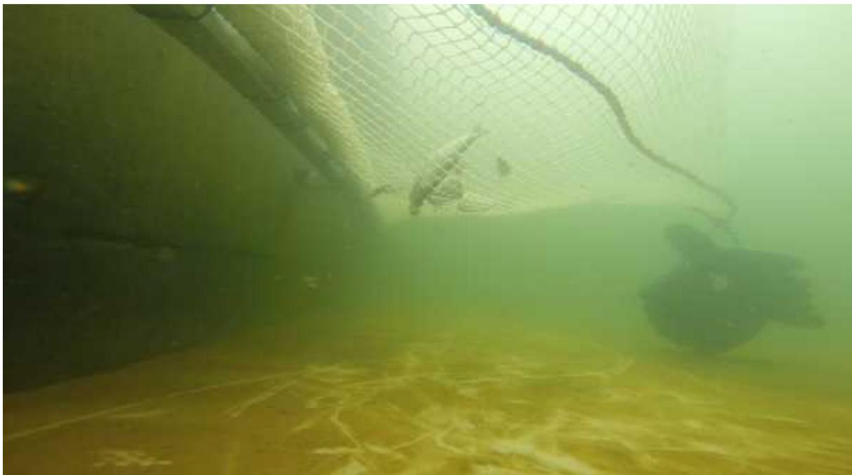
Figure 8 - The base of the netting as installed without tension. Some small fish available on the base for the seal to eat.
